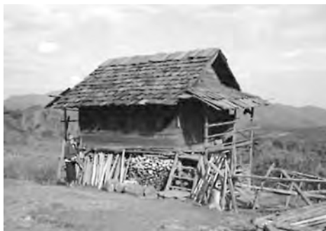
Tomb lid used as staircase landing stone, Ban Pacha (2002)
