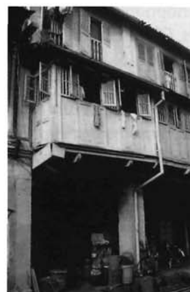
Shophouse turned into slum-additional rooms/space added to the shophouse (1980s).
